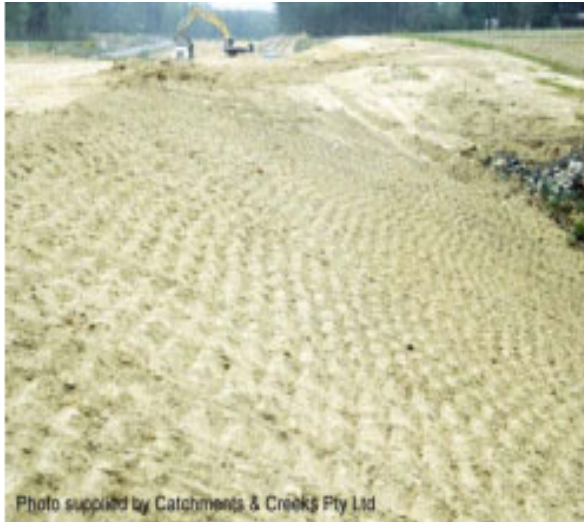
Plate 3-3 An example of a roughened slope
