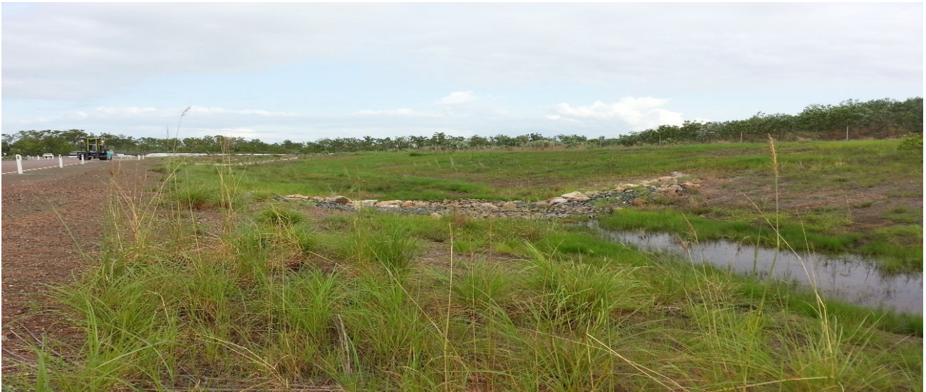
Plate 3-6 Example of Rock Check Dam and Rock Dissipater
