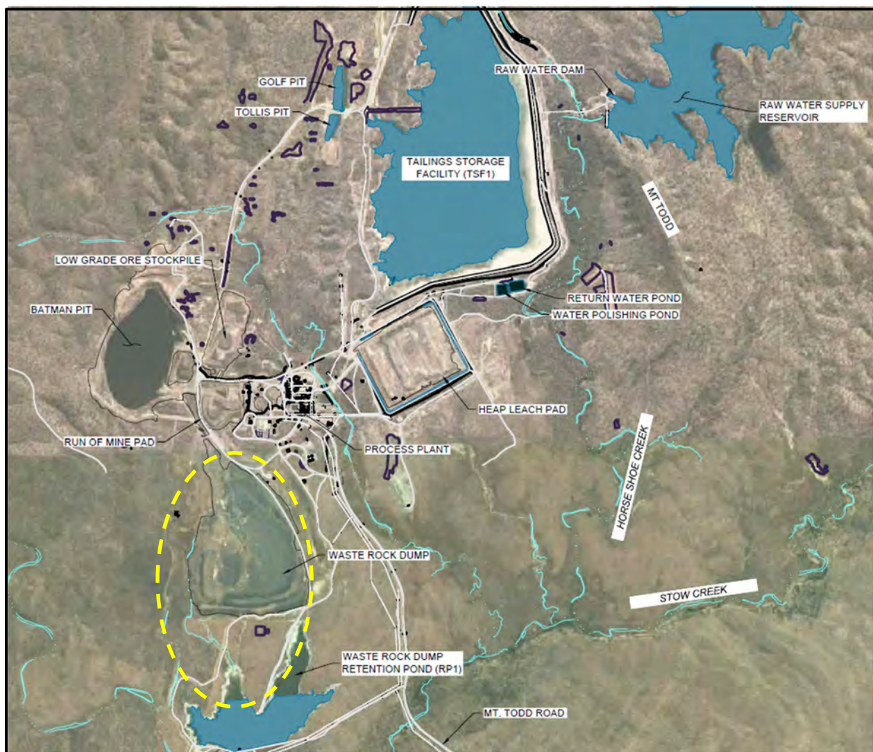
FIGURE 2.1: MT. TODD SITE – CURRENT CONDITIONS (TETRA TECH, 2018)
