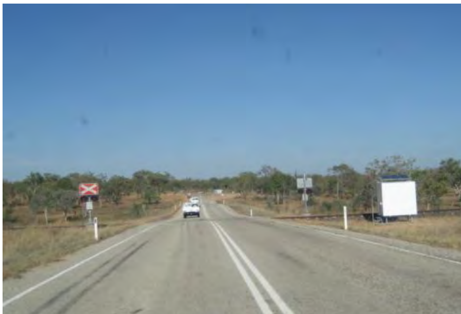
Figure 2-9 West view of Edith Falls Road Level Crossing. Stuart Highway Intersection in the background
