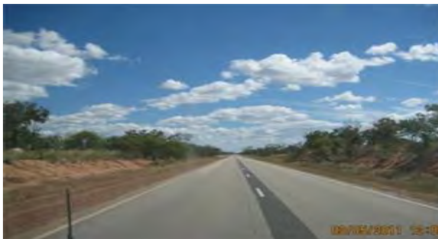
Figure 2-1 Two Lane Two Way Cross Section of Stuart Highway near Edith Falls Turn off
