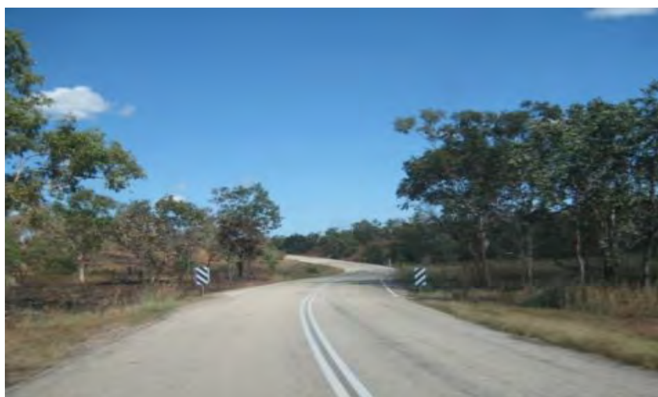
Figure 2-2 Two Lane Two Way Cross Section of Edith Falls Road with Creek Crossing
