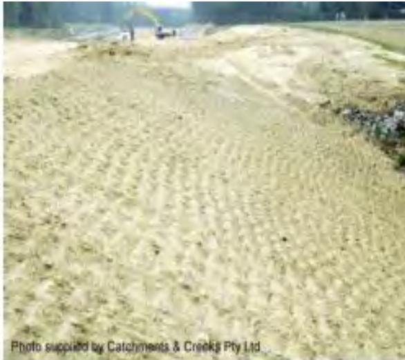
**Plate 3-3** An example of a roughened slope
