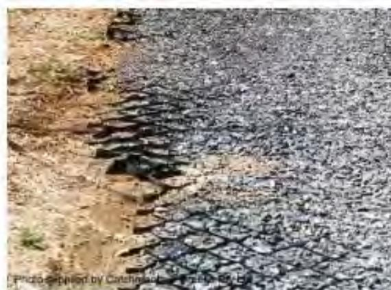
*Plate 3-2 An example of cellular confinement system used to retain soil and assist in the establishment of grass*
