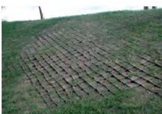
*Plate 3-1 An example of cellular confinement system used to restrict gravel movement on a carpark.*
