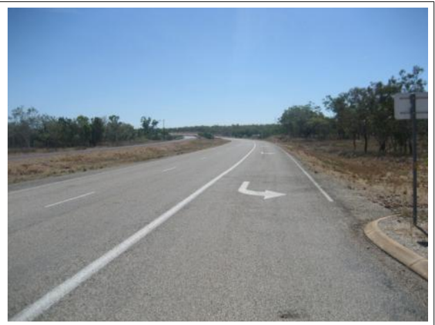
Plate 18-10 Sight Distances at the Stuart Highway / Edith Falls Road Intersection, View to north on Stuart Highway
