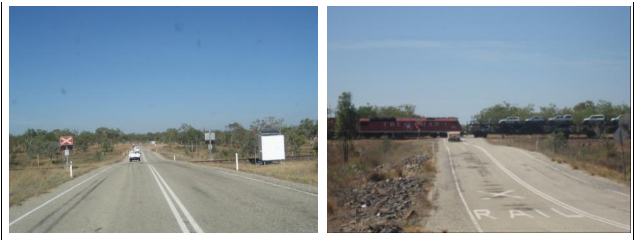
Plate 18-13 Edith Falls Road Level Crossing, View to West
