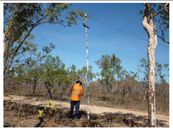
Plate 15-4 Oppenheimer Pole in Good Condition
