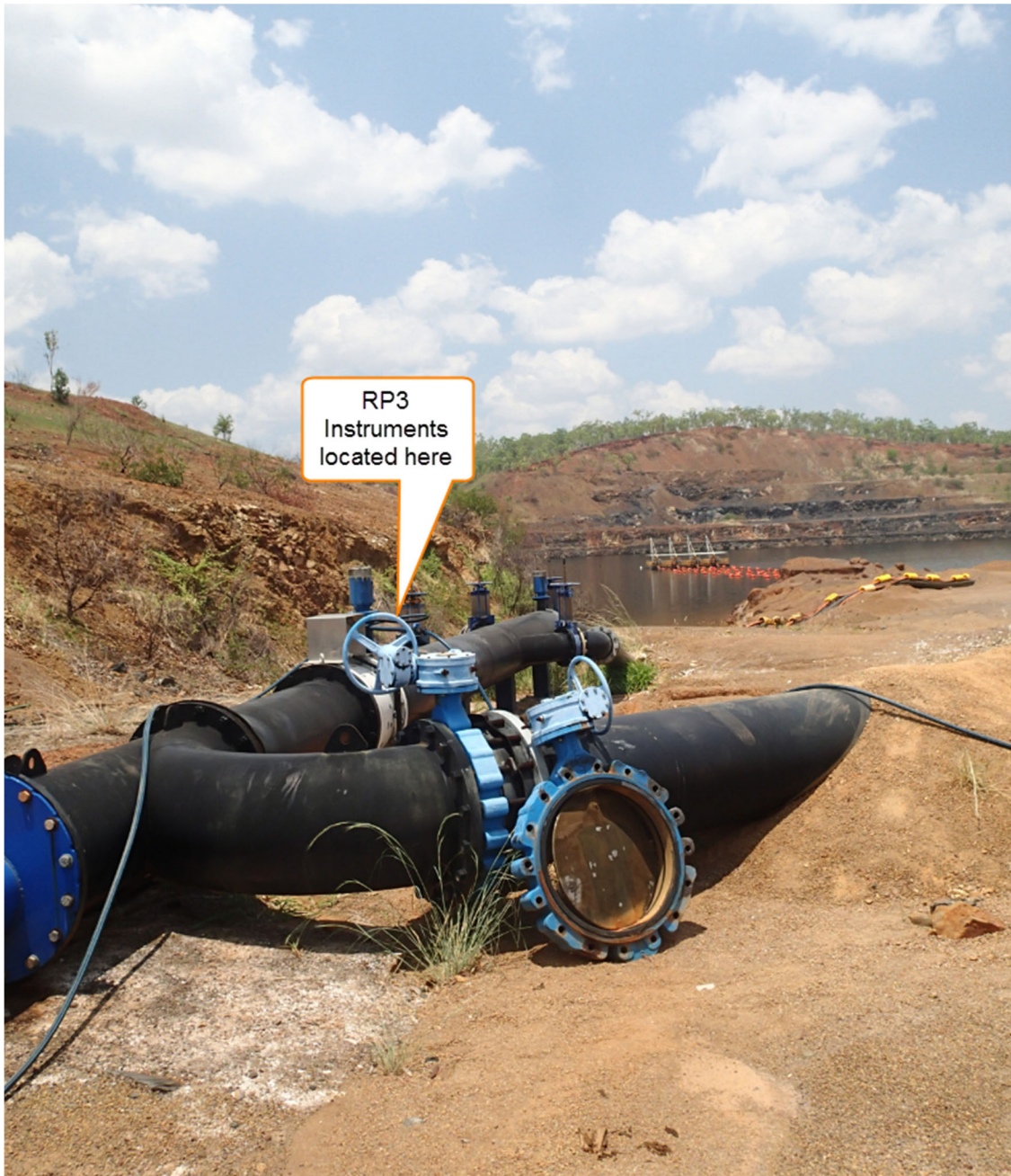
Figure 3-1 Batman Pit in-line water quality monitor
