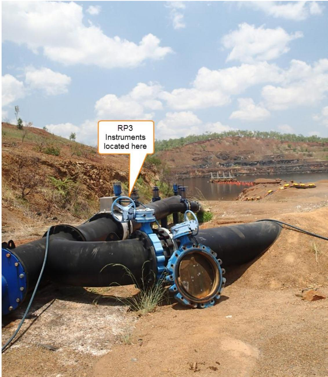
**Figure 3-1 RP3 in-line water quality monitor**
